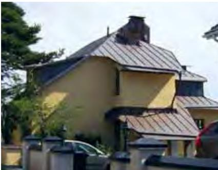
**Replacement of the failed galvanized tin roofs on this distinctive house with beautifully detailed copper has added a new dimension to its unique design.**
